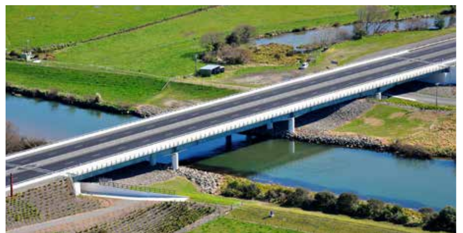
Kaituna River Bridge (TEL) Project
