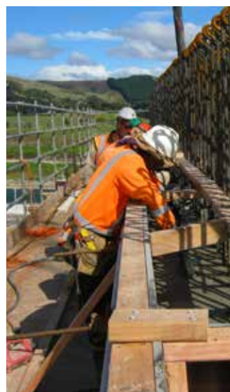
Kaituna River Bridge (TEL) Project
