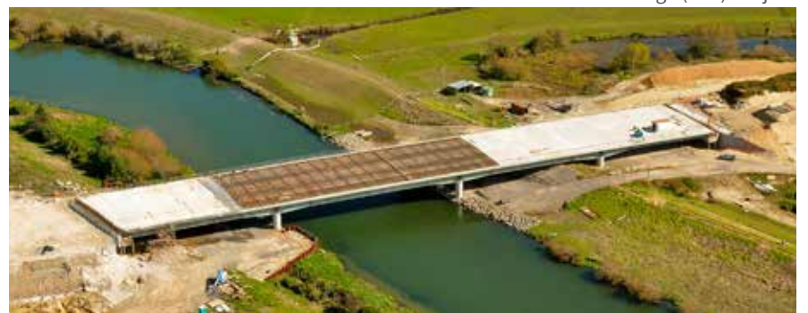
Kaituna River Bridge (TEL) Project
