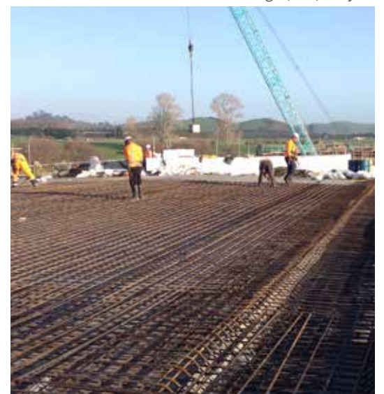
Domain Road Bridge deck construction
